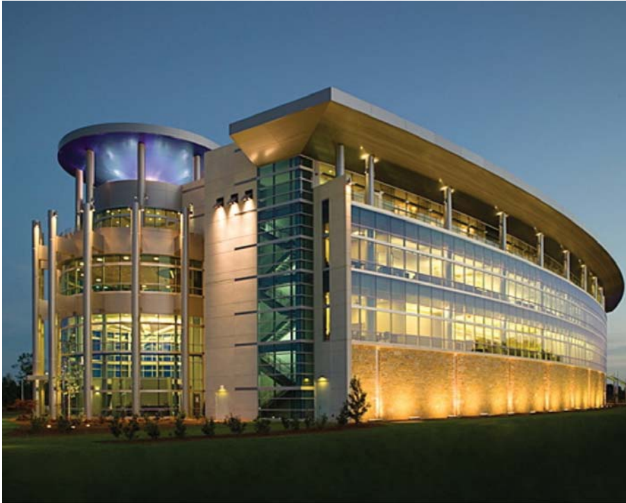
Hubbell Lighting Solutions Center, LEED Silver (Image courtesy of McMillan Smith Partners)
